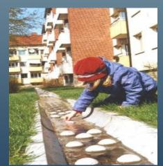
In the new storm water system, 70% of all rainwater from rooftops and other impervious surfaces is collected from gutters and channelled through canals, ditches, ponds and wetlands before finally draining into a traditional closed sub-surface storm water system. (Photo: John Dolocek, City of Malmö)
