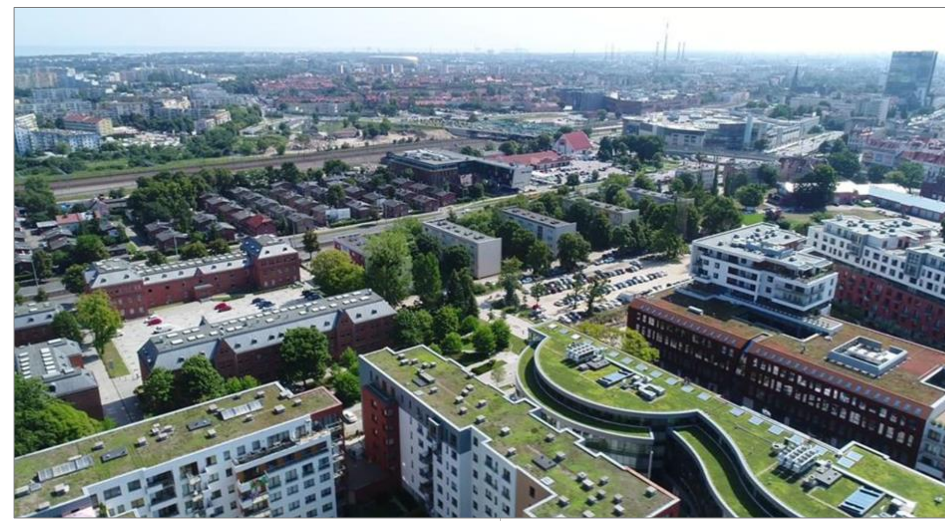
Green infrastructure Gdansk (Poland)
