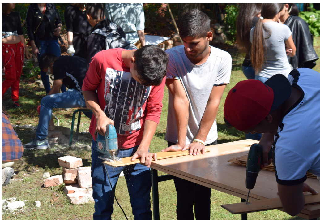
Community building during the Intensive Study Program in Dr. Ámbédkar School
