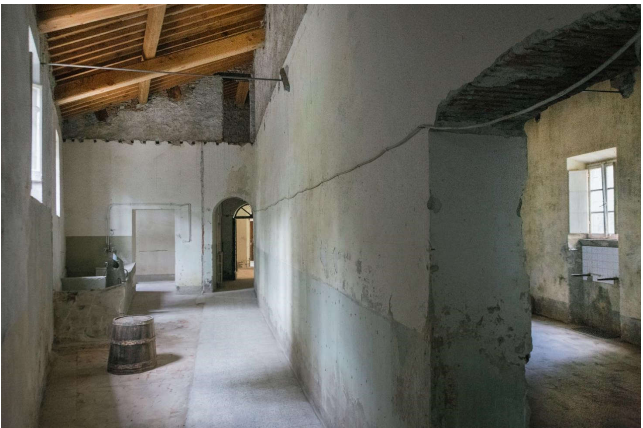
Figure 16 – A view of the internal space of the Monastery of Vicopelago.
