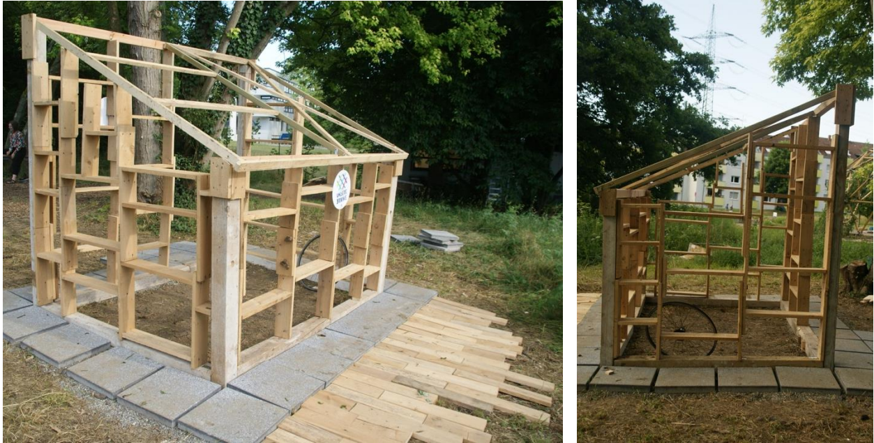
Figure 51 Finished design of the greenhouse. Photo by Ellen Fetzer.
