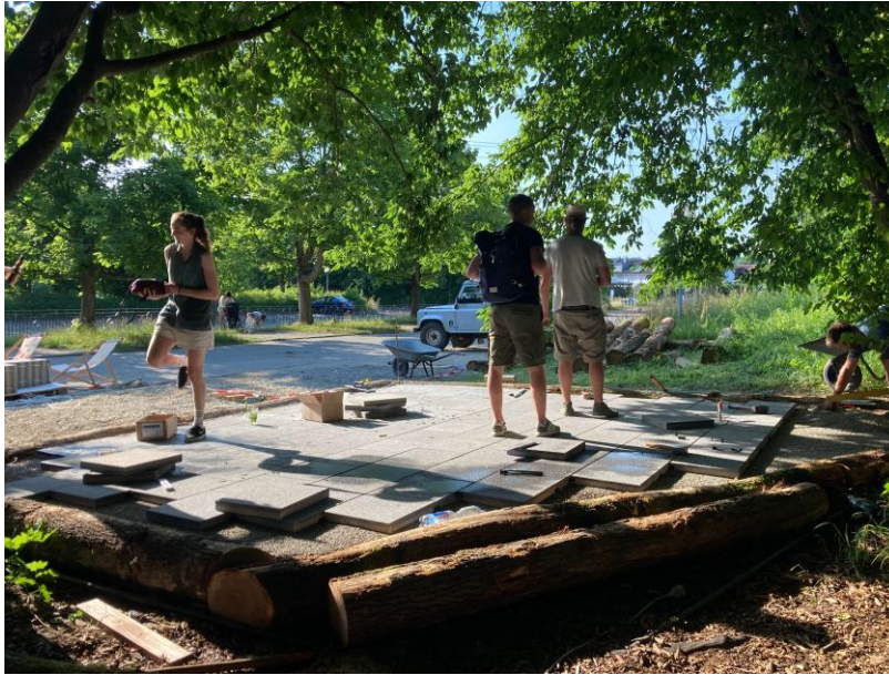
Figure 24 Terrace Construction. Photo: Karsten Michael Drohsel.
