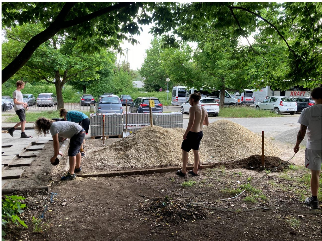
Figure 21 Starting the Terrace Construction project. Photo by Karsten Michael Drohsel.
