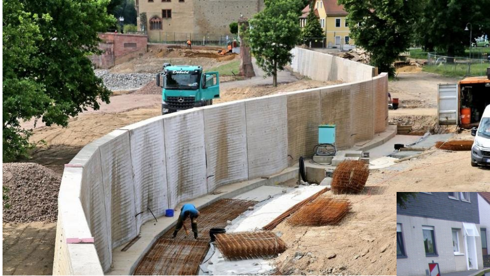
Flood protection wall in Grimma, Saxonia, source: bild.de
