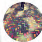
COLORING THE PAVEMENT IN SEMI-OPEN SPACE
