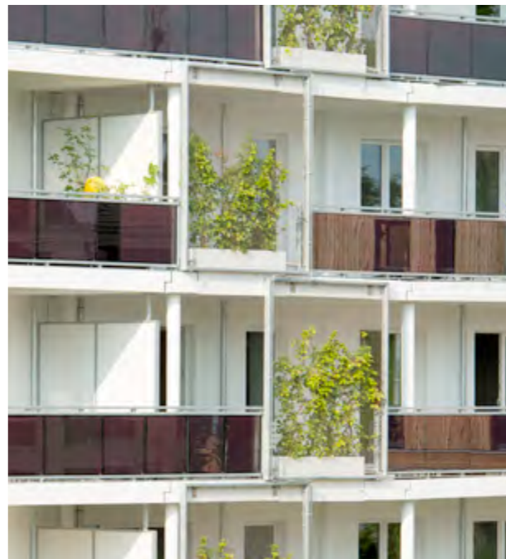
Constructive combination of PV and facade-/roof-greening (back-ventilated curtain facade with solar-panel facade based greening-system / Curtain-facade with integrated solar-modul and ground based greening (climbers) / extensive roof greening (© Nicole Pfoser, 2013)
