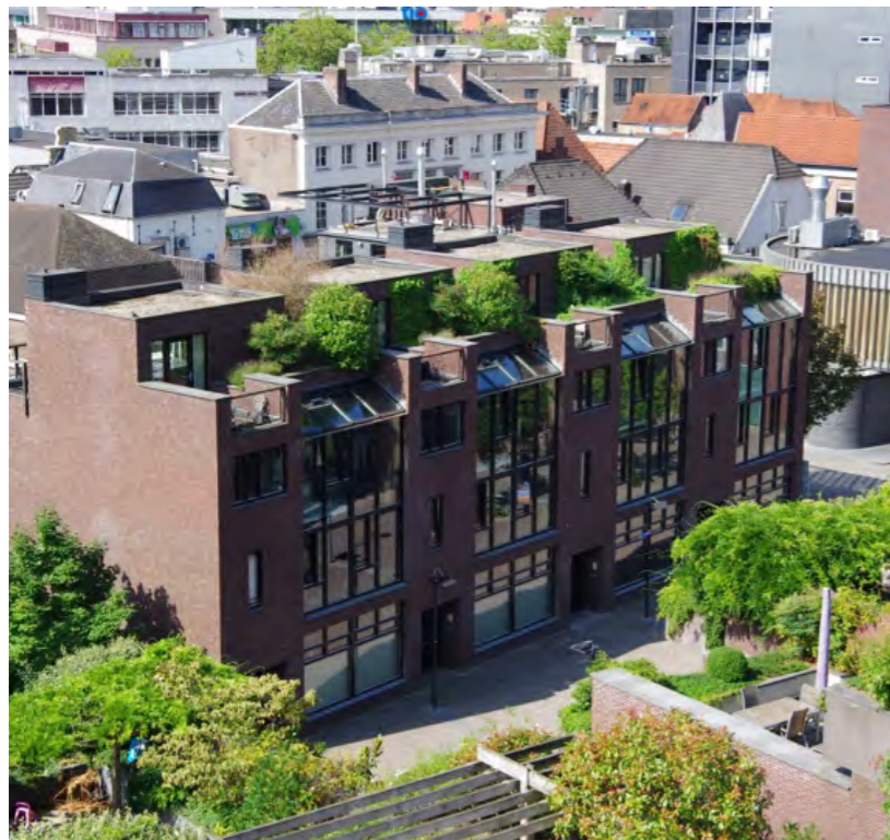
Roof gardens in Eindhoven photo: Nicole Pfoser 2013)
