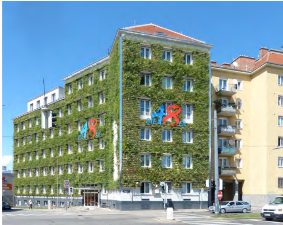
MA 48, Wien (photo: Nicole Pfoser 2012) 50% reducing heat loss of non-insulated walls (GrünStadtKlima)
