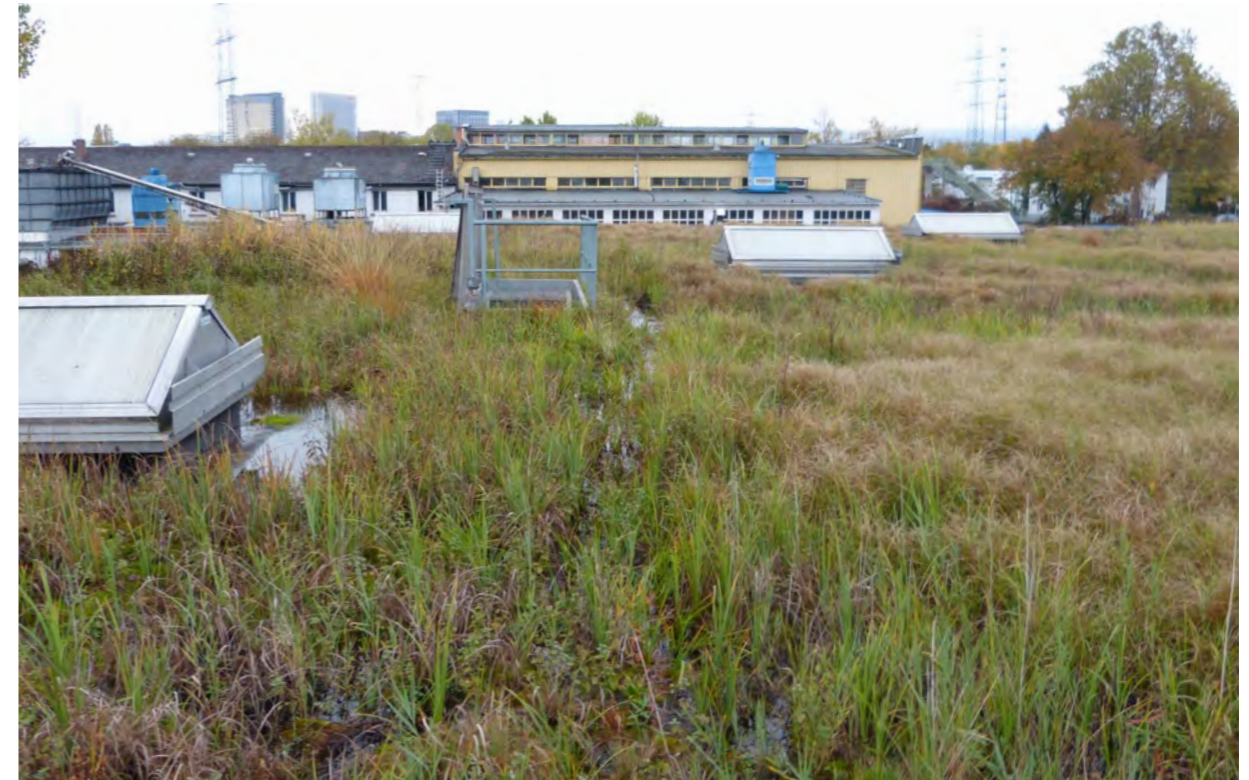
Green roof for retention and process cooling Kelterei Possmann FFM (photo: Nicole Pfoser 2012)
