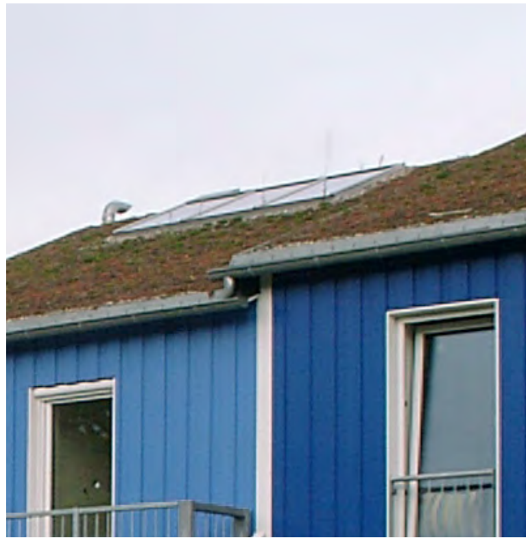
left: collectors in combination with a green roof, south orientated, Passivhaussiedlung Hannover Kronsberg (Feist, W. et al. 2001) / right: Sustainable redevelopment with solar thermal energy (photo: Markus Bachmann, Samba), www.allianz-pro-nachhaltigkeit.de
