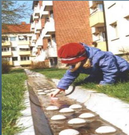
In the new storm water system, 70% of all rainwater from rooftops and other impervious surfaces is collected from gutters and channelled through canals, ditches, ponds and wetlands before finally draining into a traditional closed sub-surface storm water system. (Photo: John Dolocek, City of Malmö)
