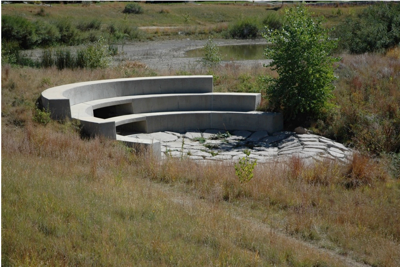
Stormwater outlets and sedimentation area. Note the use of the recycled runway paving. Photo: Austin, 2013.
