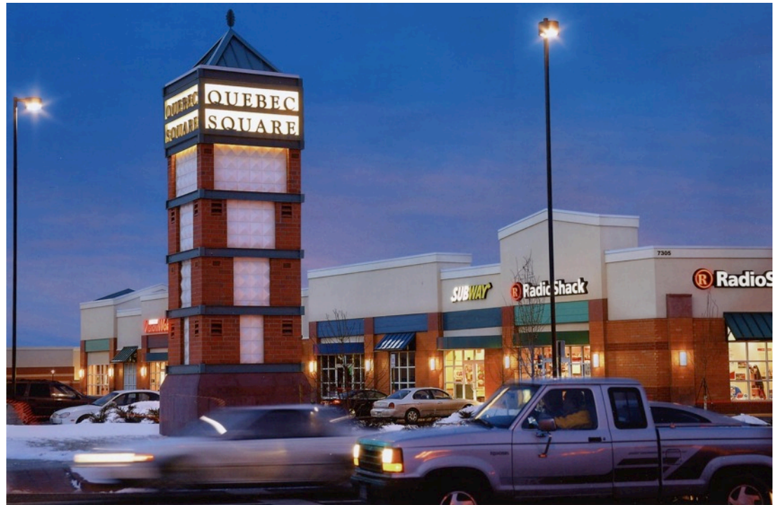
Quebec Square Regional Shopping. Photo: Forest City Enterprises Inc.
